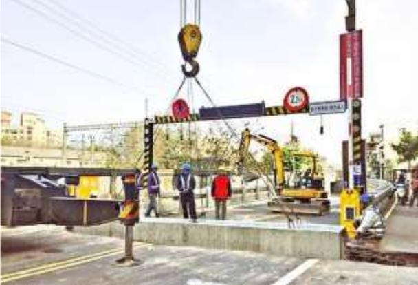
A photograph of a construction site for drainage improvement. A large crane is lifting a heavy concrete structure into place. Workers in safety gear are visible on the site.                                                     |
